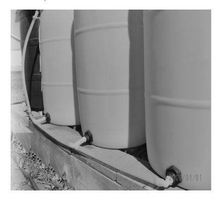
Rain Barrel system. It was a bit of a challenge to insert the connectors at the bottom with the only access being the 6" hole in the top but tips from the internet helped. A tool that is used to pick up garbage might work. If it has been a while since we've had a rainfall, divert the rain into several 5 gallon buckets until the water runs clean. To prevent algae from forming in the barrels they should be covered to protect them from the sun.
